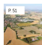
P. 51 Surplus heat integrated into district heating
