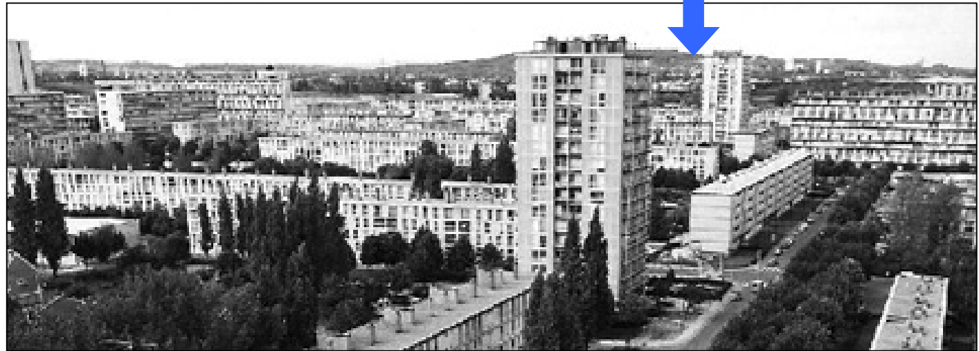
Large housing estate in Sarcelles 1955-1975 – 12,000 units (2/3 social)
