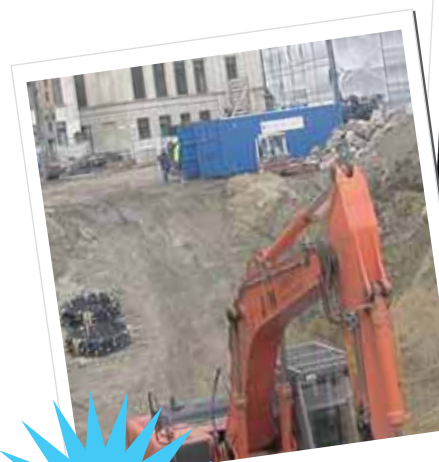
Parking Ramen fase 1
